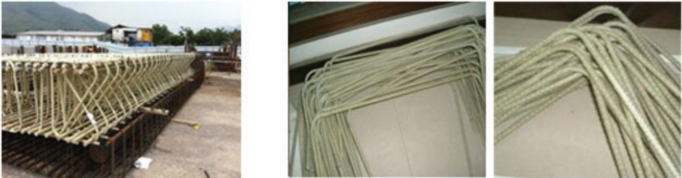
Fig. 6.1 Bending of GFRP bars ( http://www.pulwellpultrusions.com )
