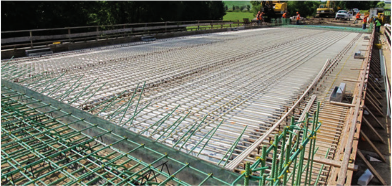
Fig. 2.1 Bridge Panel Construction Using GFRP Bars (www.tuf-bar.com)
